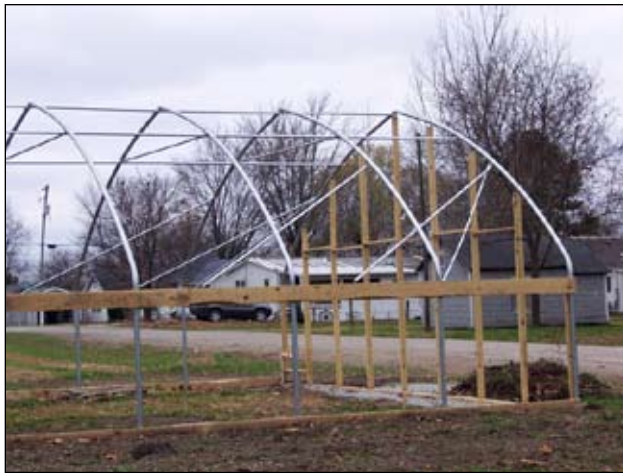
High tunnel at Lowery City.
