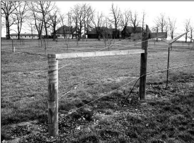
Fig. 6-5. Single span brace assembly
