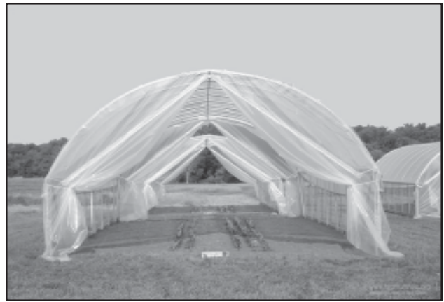
Relatively low cost plastic covered high tunnel structure at the Eastern Kansas Horticulture/Forestry Research and Education Center.
