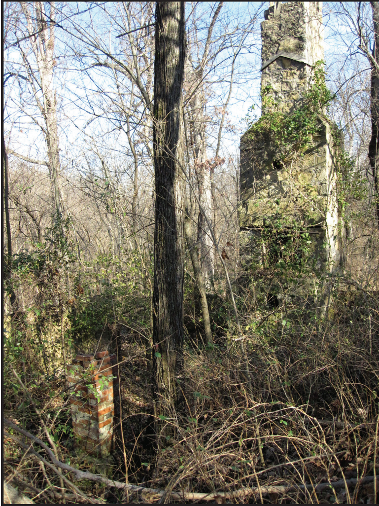
Ruin of Superintendent's Timber Home — 2013
