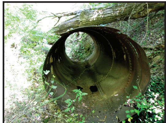
Massive Pipe – Possibly from Laundry's Boiler — 2013 Located Along the Creek Below Broken Dam Courtesy of Timothy Stanton
