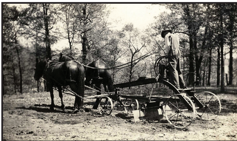
Grading a Road — 1934 Courtesy of The State Historical Society of Missouri
