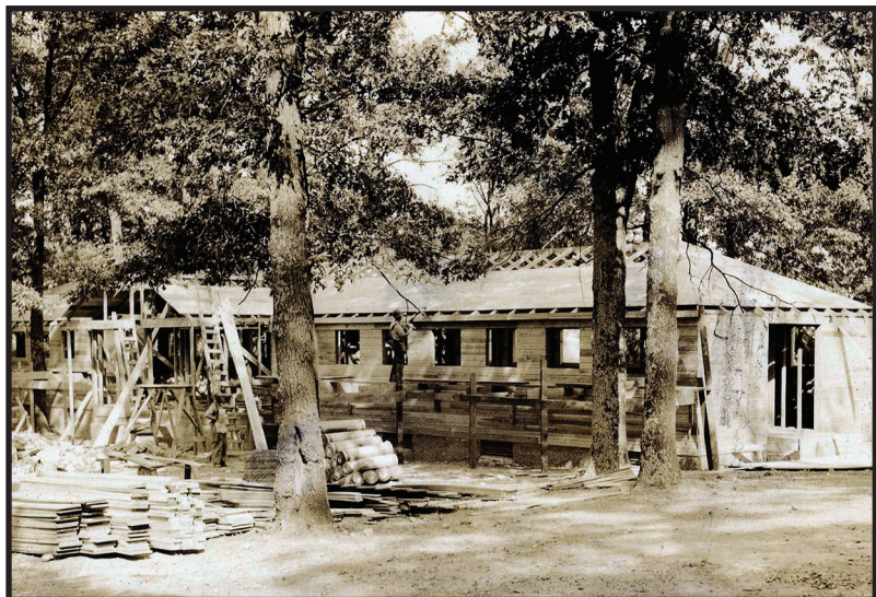
Dormitory No. 3 Under Construction — 1934 Courtesy of The State Historical Society of Missouri
