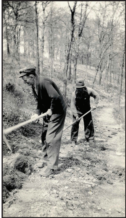
Building a Road — 1934 Courtesy of The State Historical Society of Missouri
