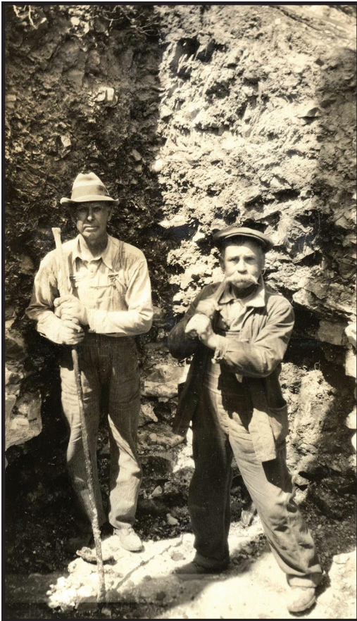
Excavating a Septic Tank — 1934 Courtesy of The State Historical Society of Missouri
