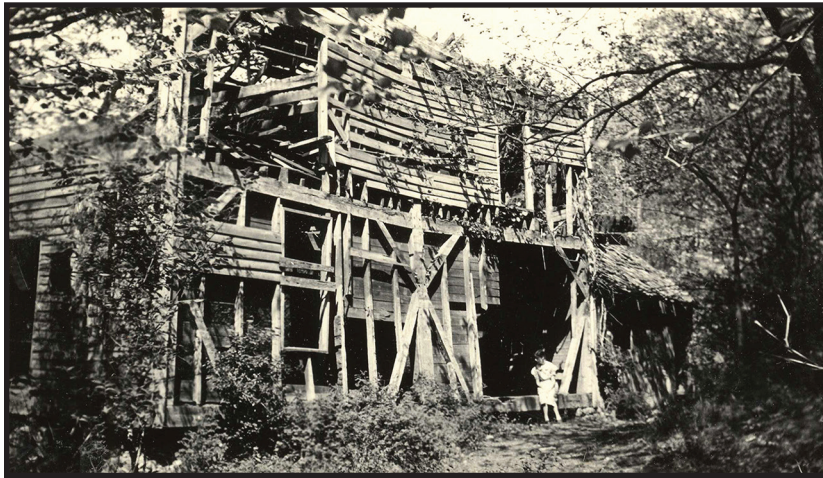
Dilapidated Ritter Mill — 1934
